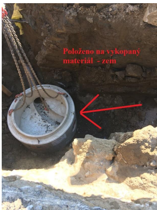
Obr. stoka B1 šachta 10 -3
